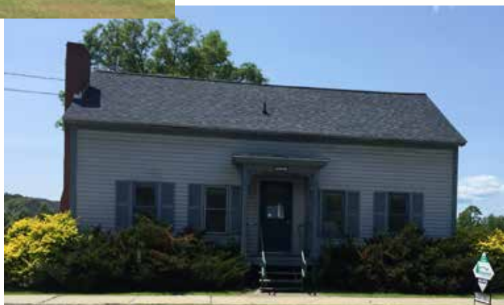
Old Hinesburg police station before transformation into Energy Futures Group building.
