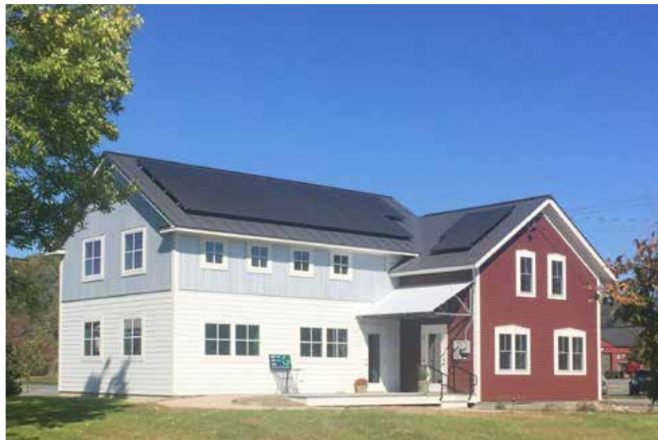
Energy Futures Group building from the south. All photos courtesy of Richard Faesy.
